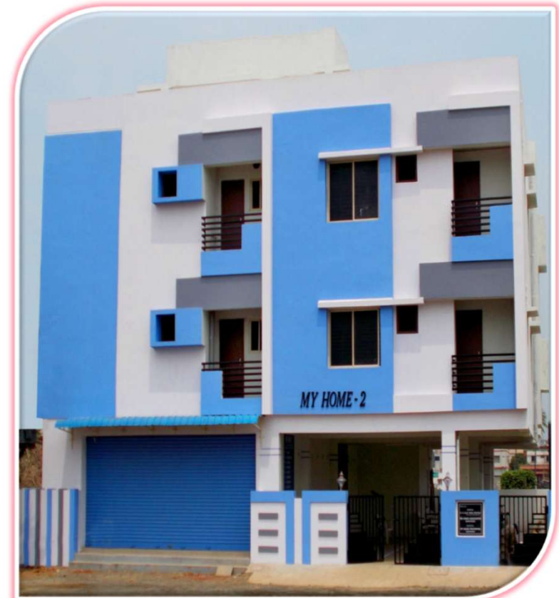
Project : Residential Apartment Area: APSP, Kakinada
