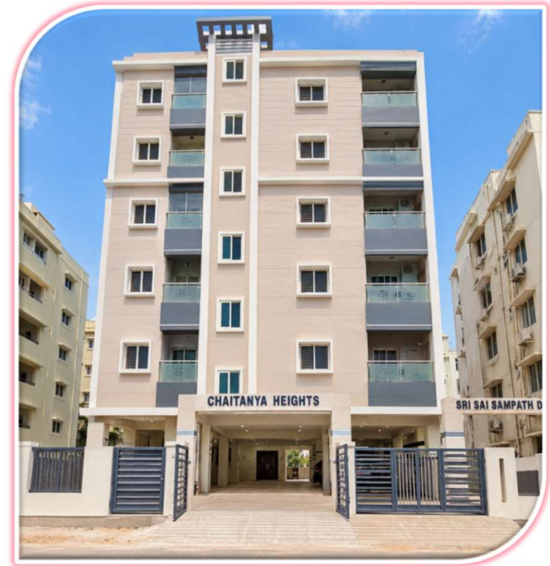
Project : Residential Apartment Area: Rajeswarinagar, Kakinada
