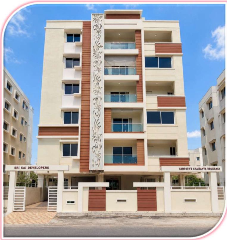
Project : Residential Apartment Area: Rajeswarinagar, Kakinada
